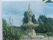
1888 TERRACOTTA ON AN IRON FRAME. IT STANDS IN FRONT OF THE PEOPLE'S PALACE, WHICH HOUSES THE CITY'S SOCIAL HISTORY COLLECTIONS
